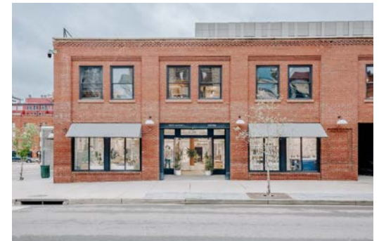
Older Commercial Building Restoration
