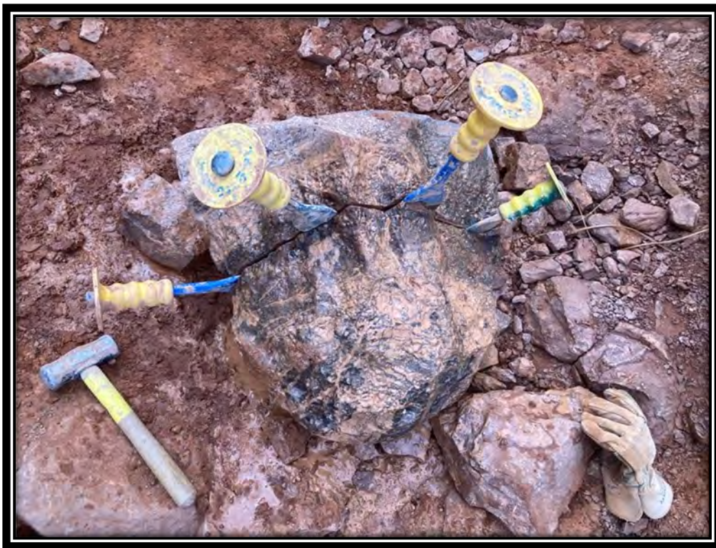
Crews learning how to safely rig rock and another example of splitting techniques that were learned on the Cathedral Rock project.
