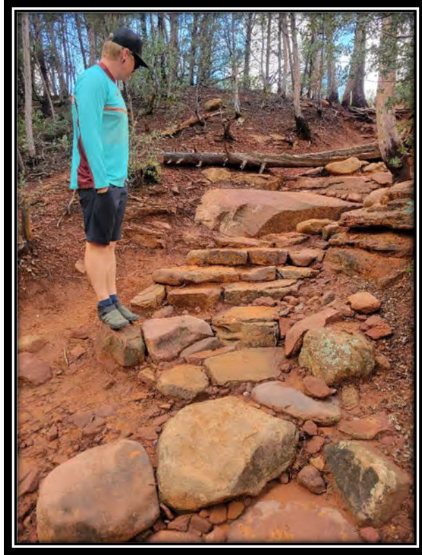
Failing rock check steps to be reconstructed near Soldiers Wash in Fall of 2023 (above). Social trails and drainage needs along Soldiers Pass trail (below).
