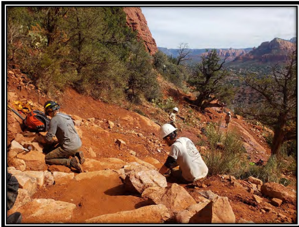
ACE Crew constructing rock check steps on Cathedral Rock trail.
