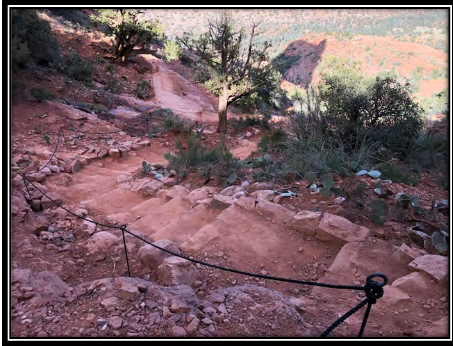
New fencing to better delineate the system trail and rock check steps to harden erosive soils.
