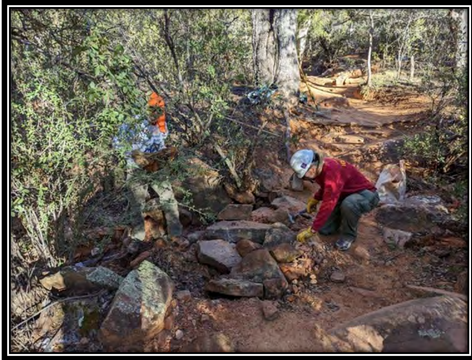
Friends of the Forest Crew building a retaining wall to fortify the trail.
