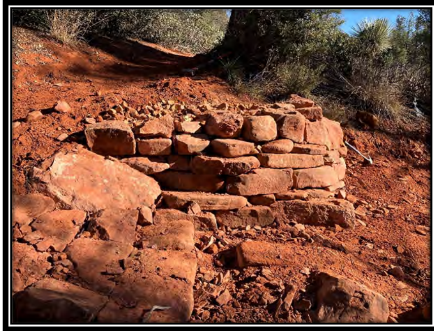
New retaining walls and rock armored ramps.
