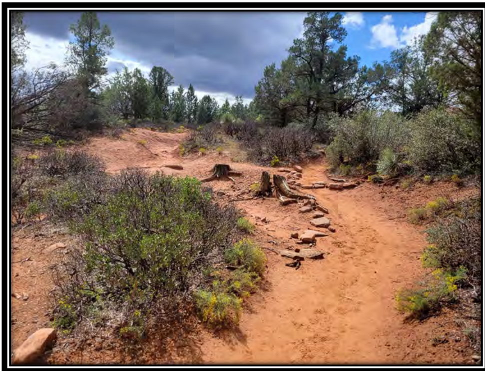
Failing rock check steps to be reconstructed near Soldiers Wash in Fall of 2023 (above). Social trails and drainage needs along Soldiers Pass trail (below).
