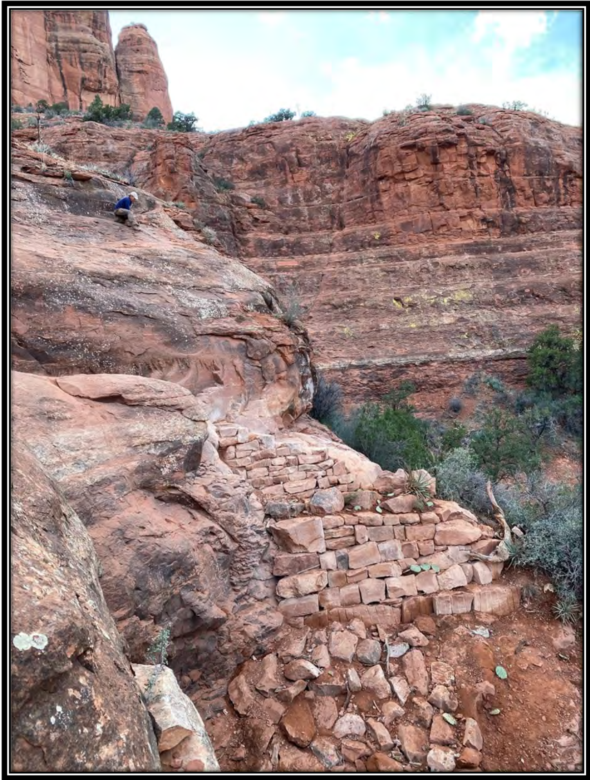
Summit to Sea Trails Specialists constructed this 30ft high retaining wall, installed check steps, and assisted with restoration of user created routes.
