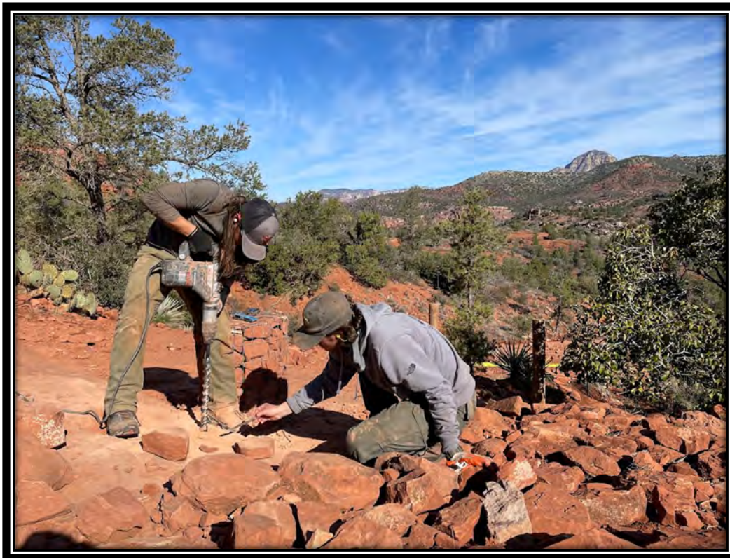
(Above) Crews constructing new checks steps and (Below) installing fencing.
