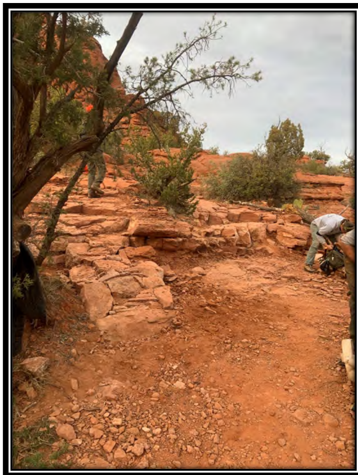
New retaining walls and rock armored ramps.
