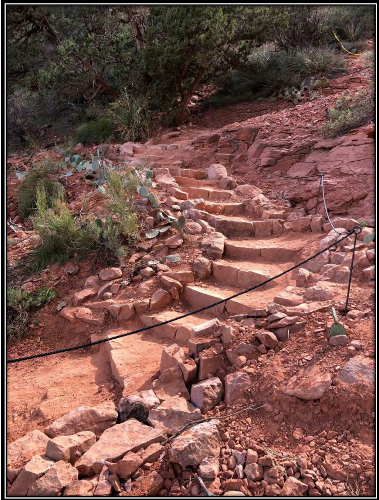
New check steps and trail delineation fencing.
