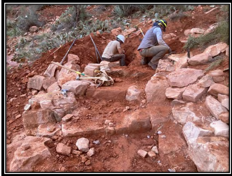
ACE Crew constructing rock check steps on Cathedral Rock trail.
