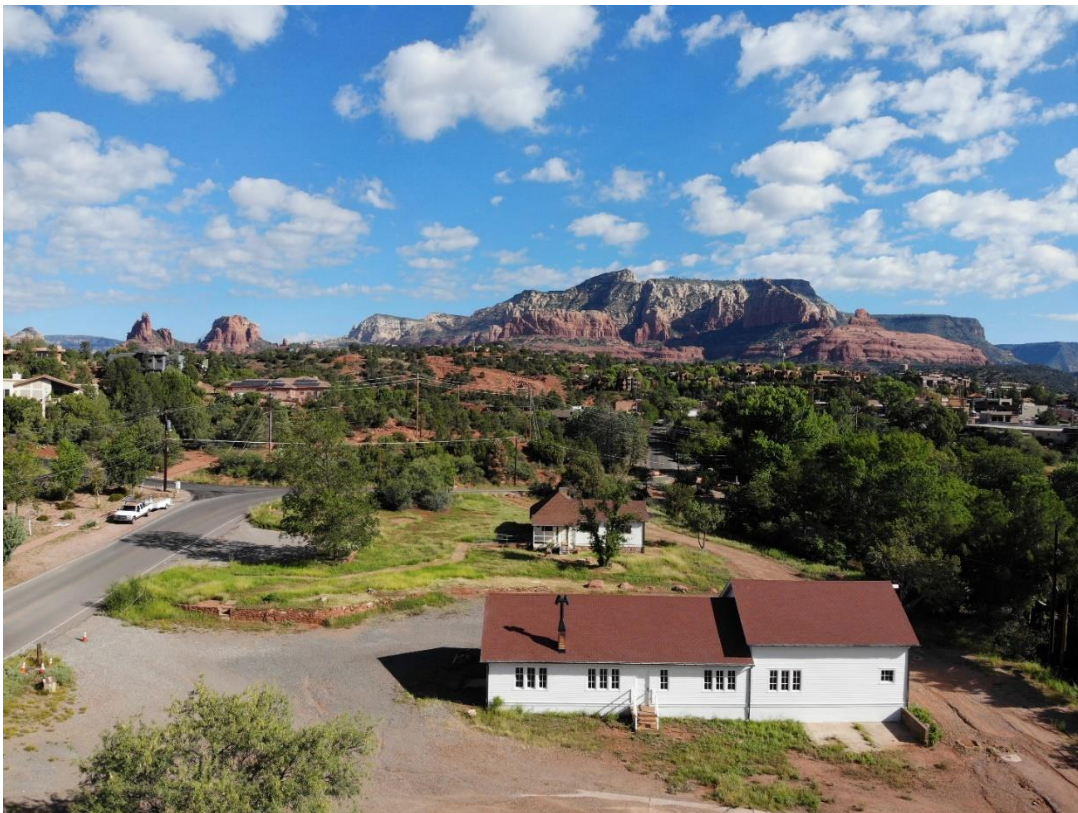
Recent drone photo of site illustrating exterior rehabilitation complete
