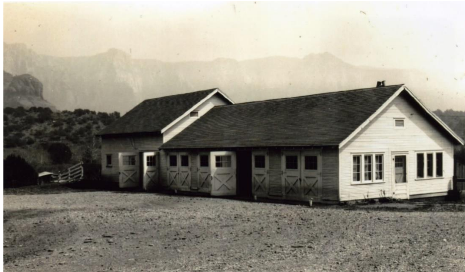
Historic photo of barn, date unknown
