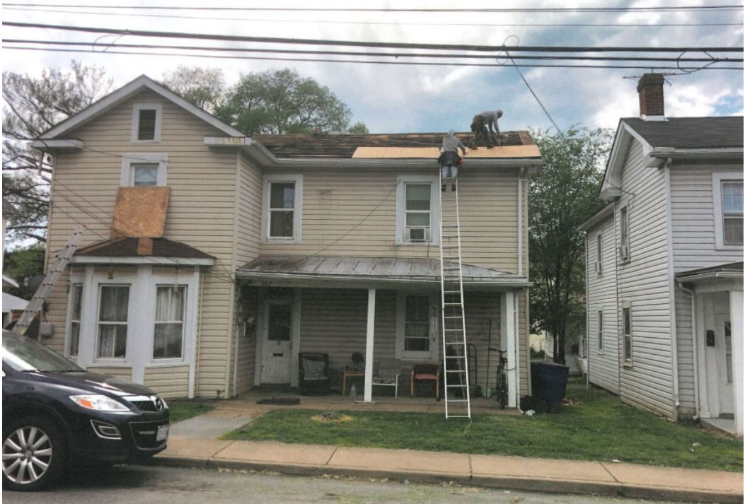
Photo 3 – view of front building elevation – after removal of metal roof
