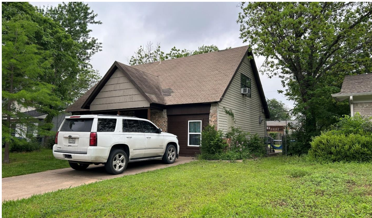
View of the converted garage from Linhaven Drive, facing southwest.
