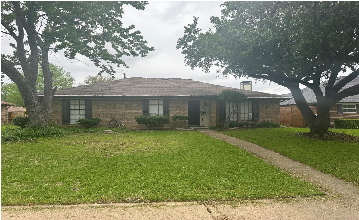
Subject property from Meandering Way.
