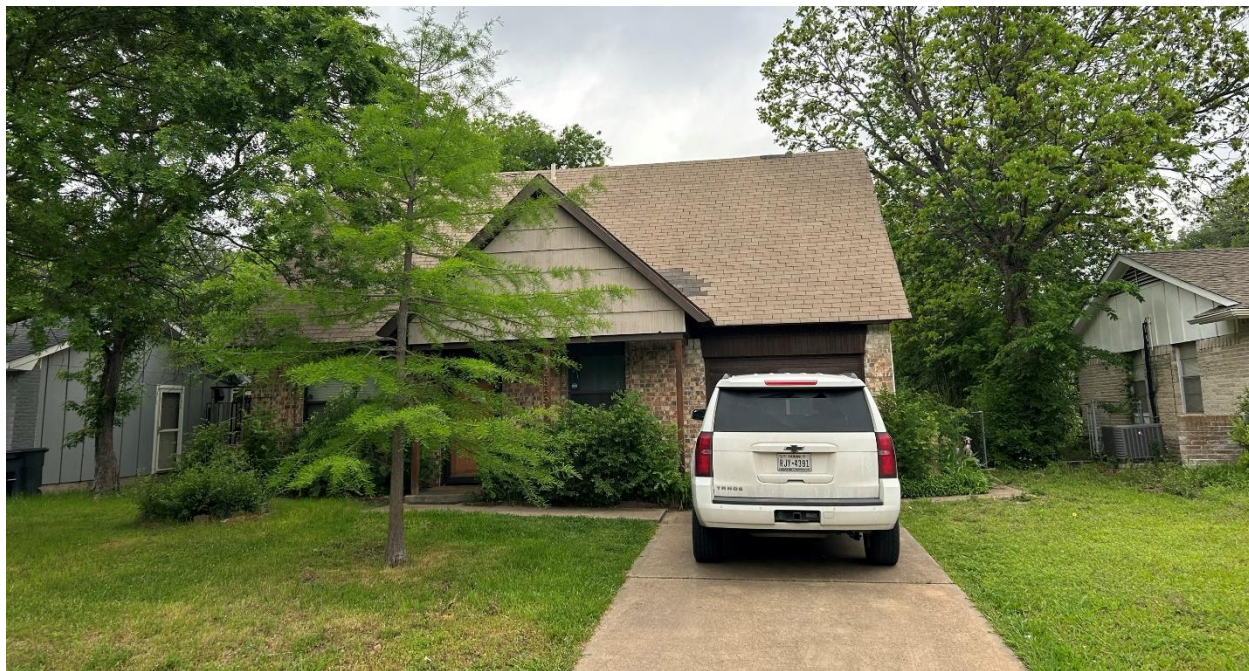
Subject property from Linhaven Drive, facing northwest.
