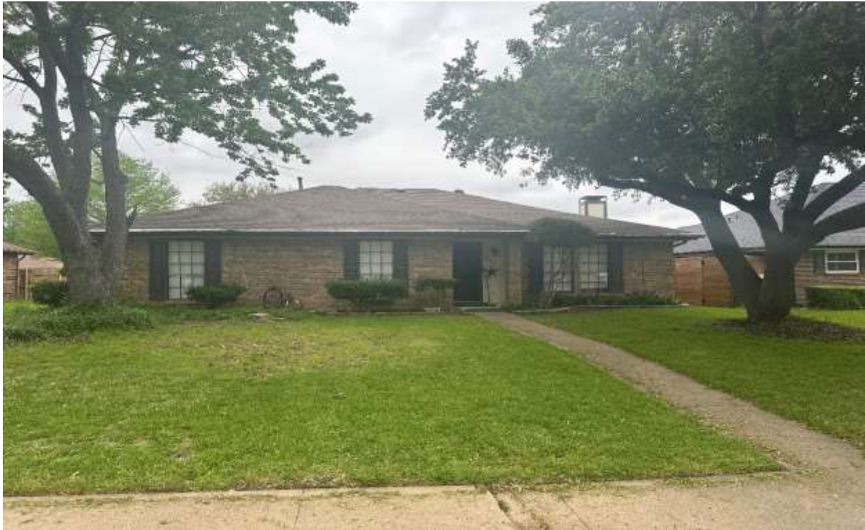
Subject property from Meandering Way.
