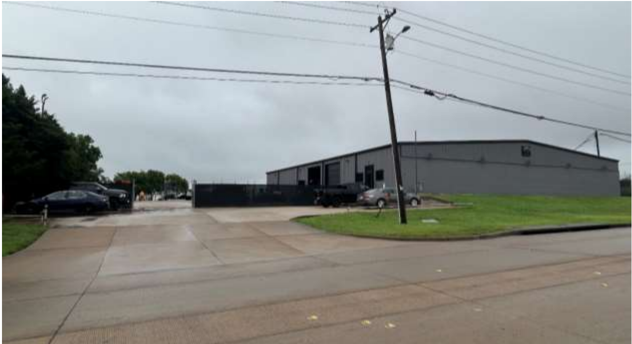
Front view of the subject property, facing South
