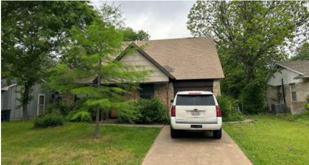
Subject property from Linhaven Drive, facing northwest.
