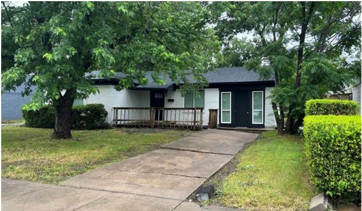
View of the converted garage from Hyde Park Drive, facing southwest.
