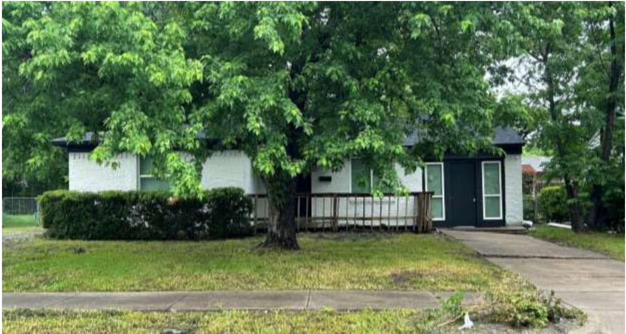
Subject property from Hyde Park Drive, facing west.
