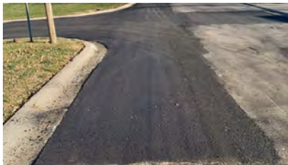
Asphalt Street Patching
