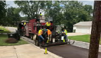
Modified Aggregate Quick Set (MAQS) Resurfacing Project
