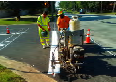
Pavement Marking Project
