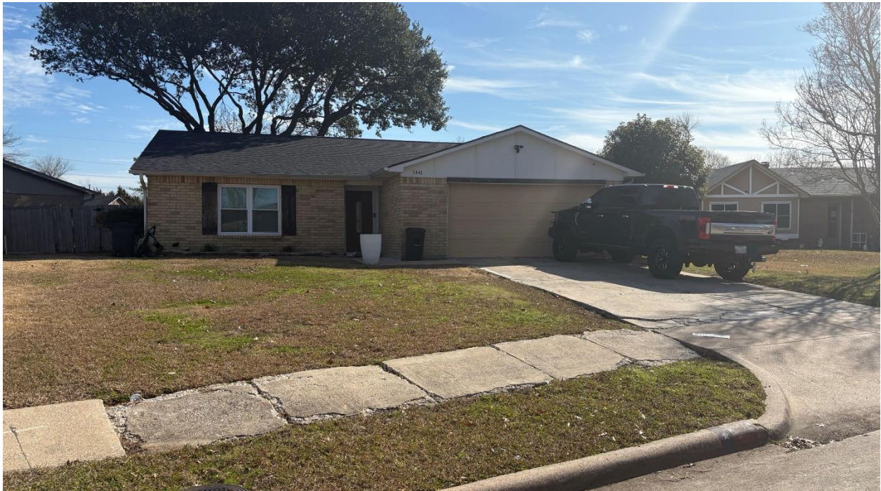
Front view of the subject property, facing east
