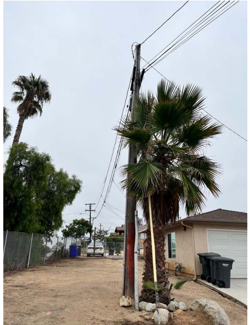
Looking south towards overhead utilities
