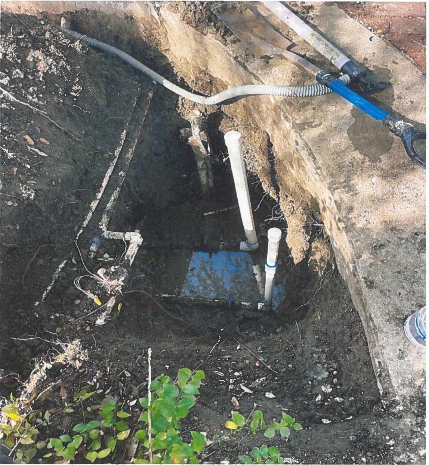
SoCo Depot Irrigation Replacement
