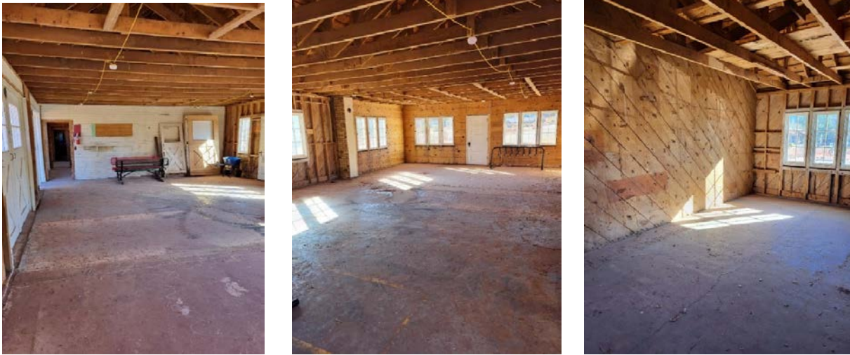
Assembly Space in Ranger Station Barn
