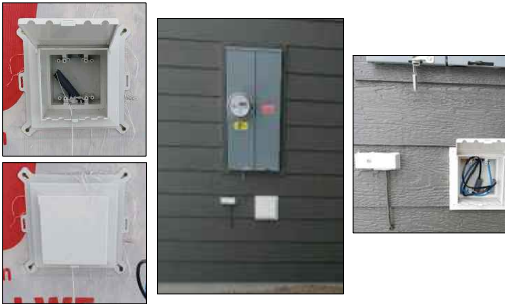
EXAMPLE 3 OF EXTERIOR COMMUNICATION WALL MOUNT
