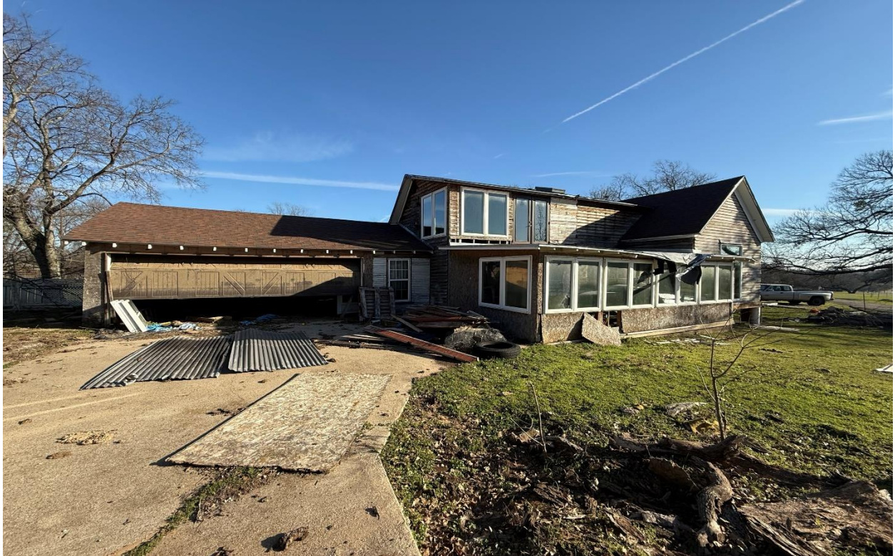
View of the garage, facing north
