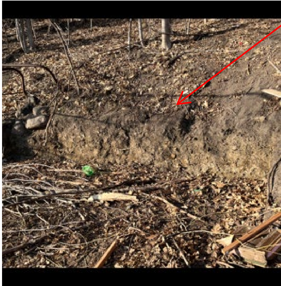
After shed demo
