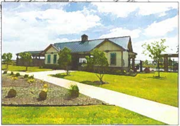
AMENITY CENTER RESTROOM BUILDING
