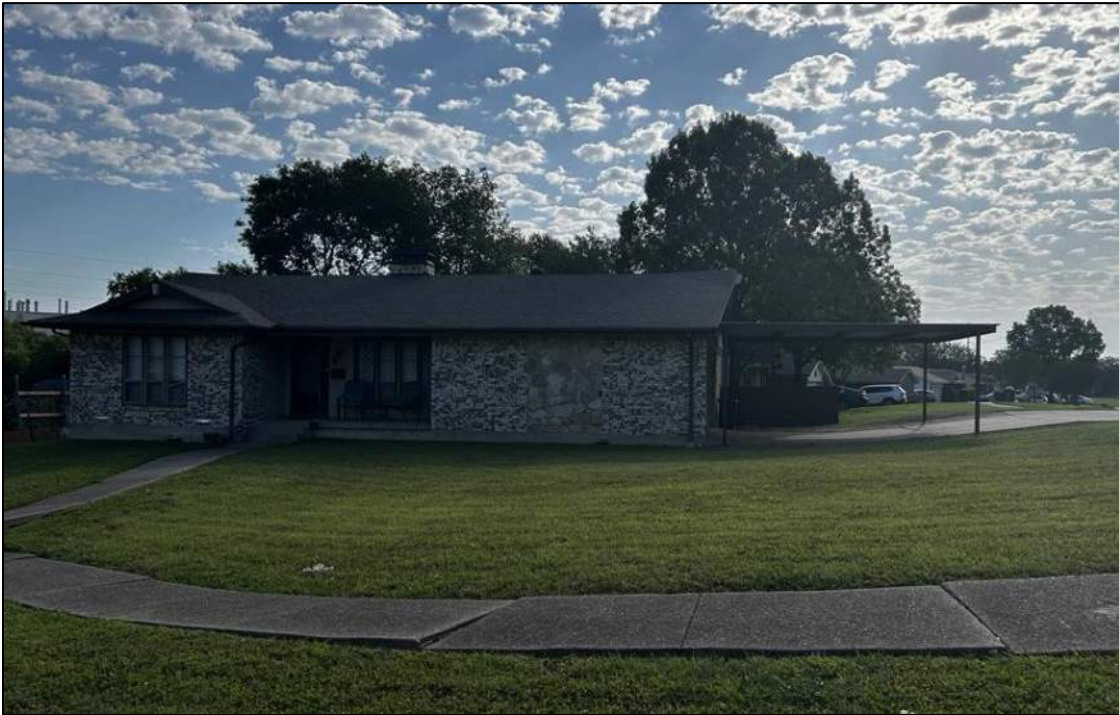
Front view of the subject property, facing east
