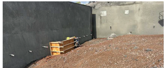
Northwest Corner of Garage - Soil Nail Wall
