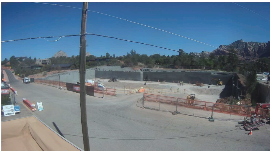
Uptown Parking Garage Site on May 19, 2025
