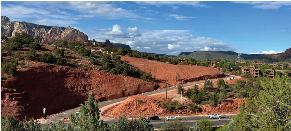
The Completed Forest Road Connection
