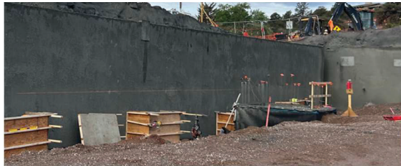
Southwest Corner of Garage - Soil Nail Wall
