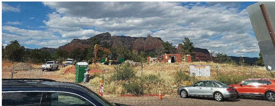
Uptown Parking Garage Site on October 10, 2023
