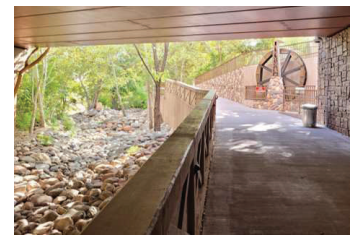
Ped Crossing at Oak Creek
