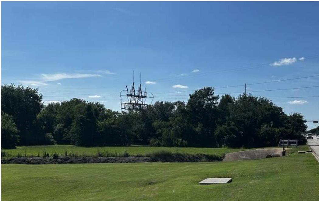
View of adjacent drainage channel, facing northwest
