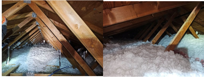
Figure 1: Before and after pictures of insulation replacement through the Home Energy Retrofit Project.
