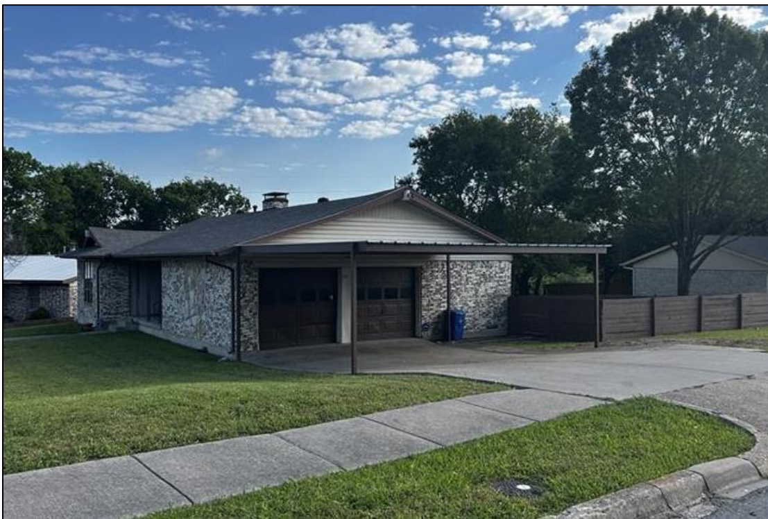
Exterior side view of the subject property, facing north
