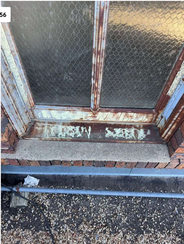
Project: The Rogers Hotel Date: Mar 17, 2025, 10:54 AM Creator: DFW AND SOUTH TX COMMERCIAL DIVISON
