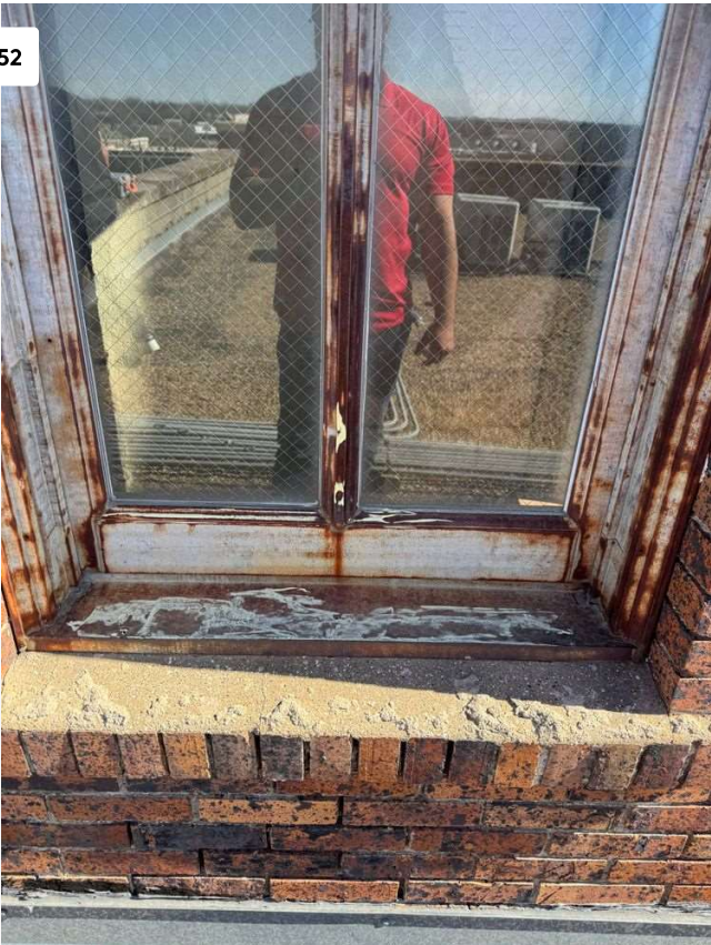
Project: The Rogers Hotel Date: Mar 17, 2025, 10:50 AM Creator: DFW AND SOUTH TX COMMERCIAL DIVISON
