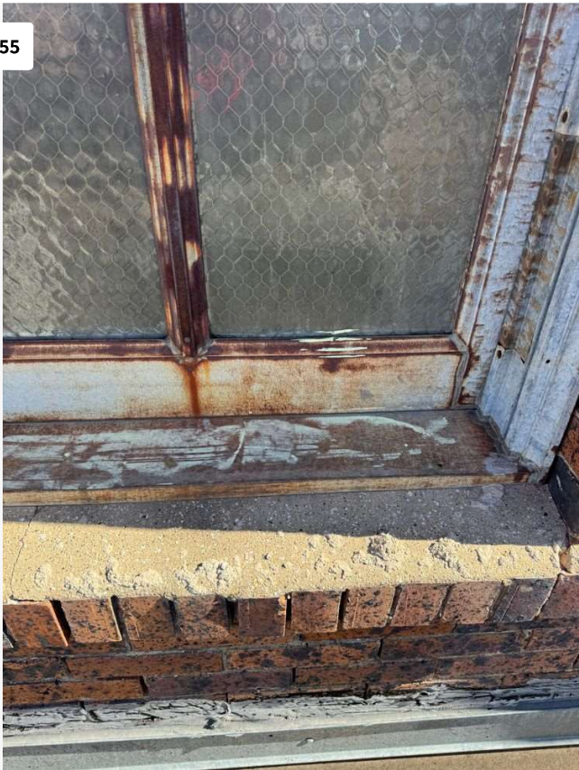
Project: The Rogers Hotel Date: Mar 17, 2025, 10:52 AM Creator: DFW AND SOUTH TX COMMERCIAL DIVISON
