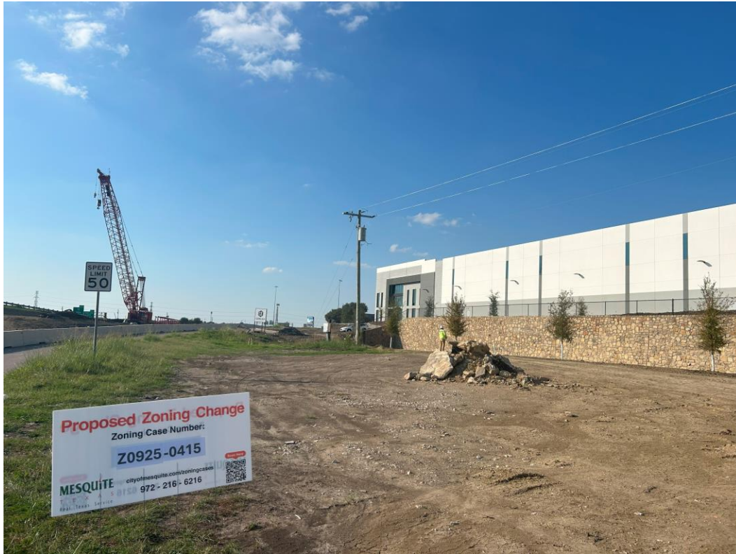
Facing north along IH-635 service road
