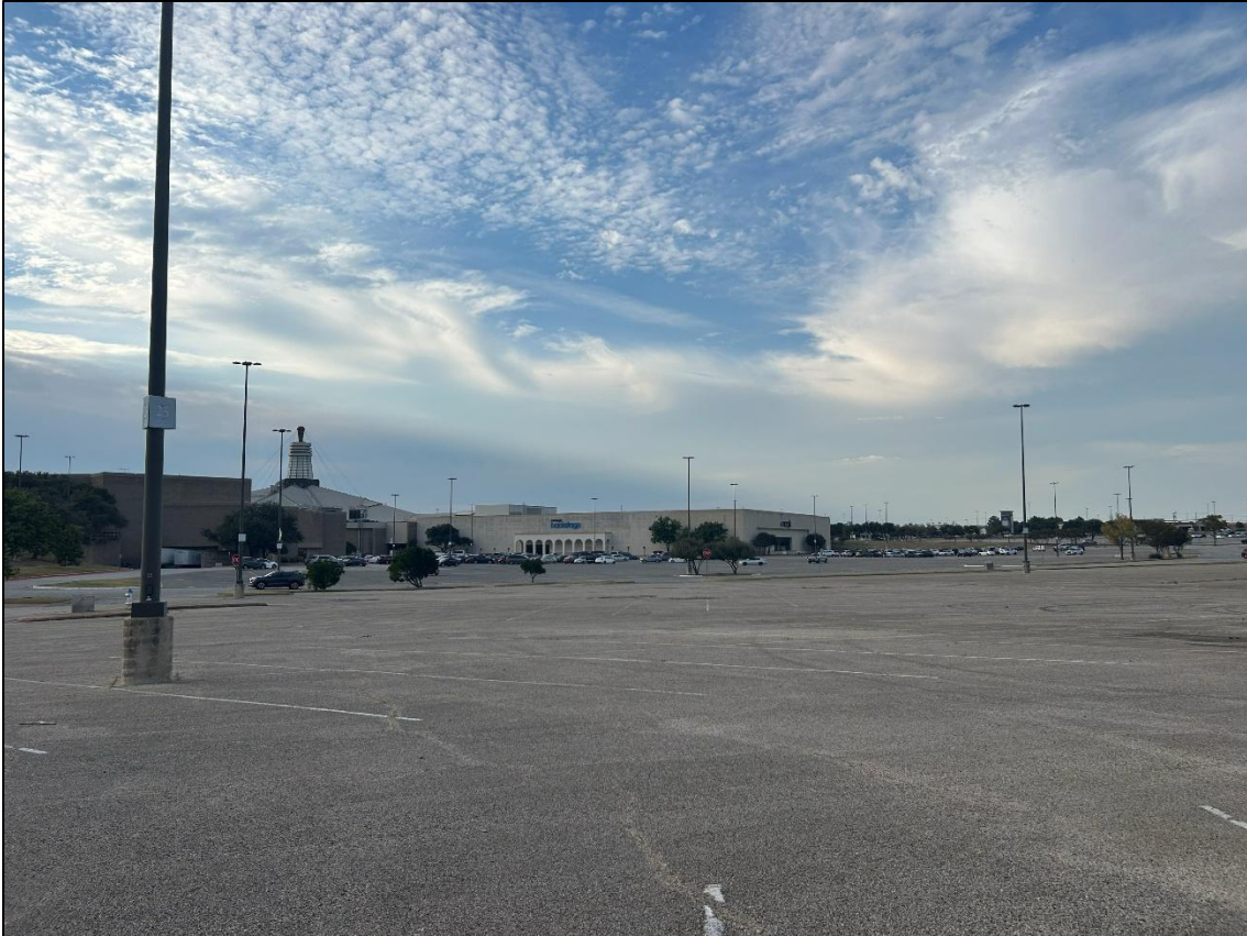
Subject property showing parking, facing north.
