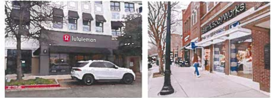
Example of ground articulation between ground floor and upper level mixed use
