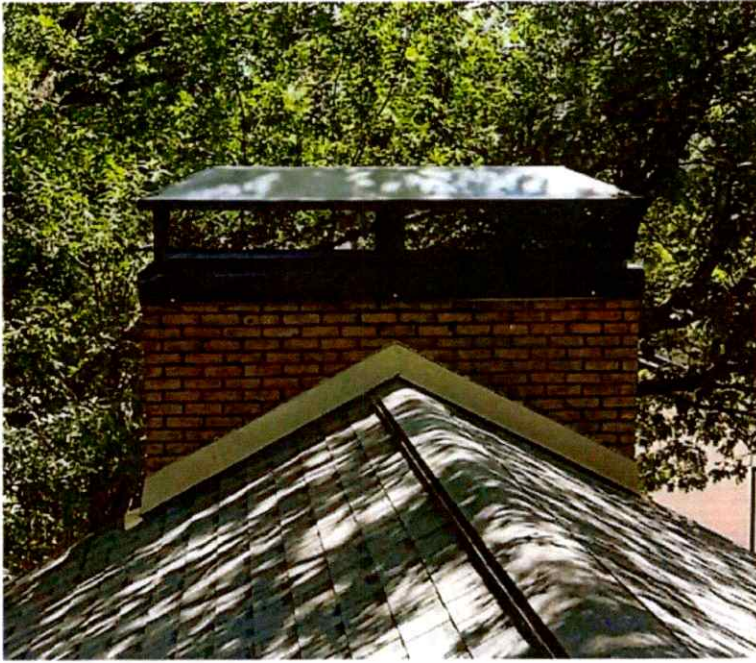
Den Chimney After
