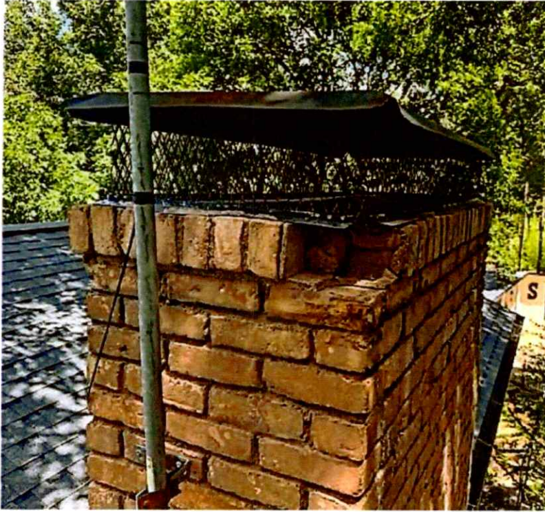
Kitchen Chimney Before
