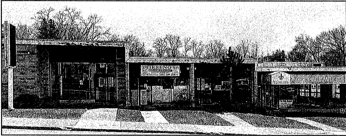
Photo 1 - Commercial building on Lot 1
