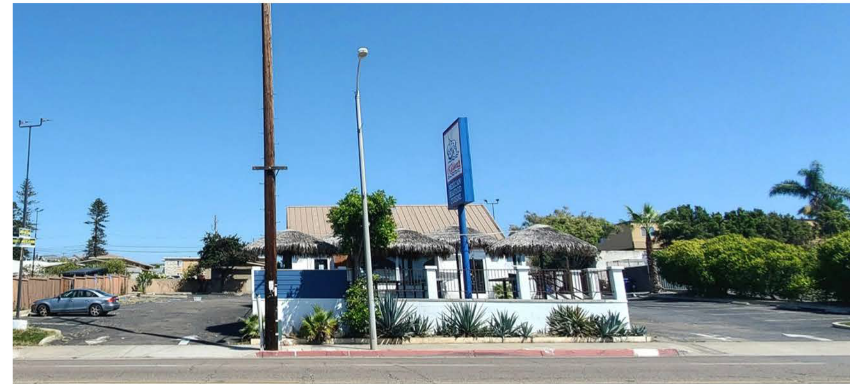
B) AREA OF WORK
