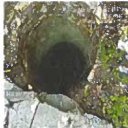
Added on: 03-18-2026 (Direct Link) Notes: exposed well
