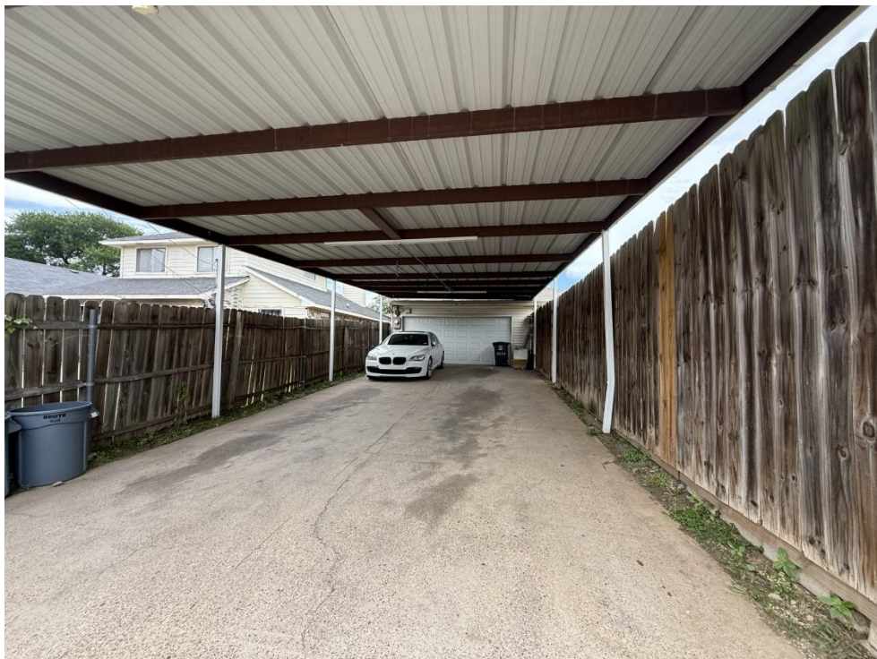
Subject property's rear carport
