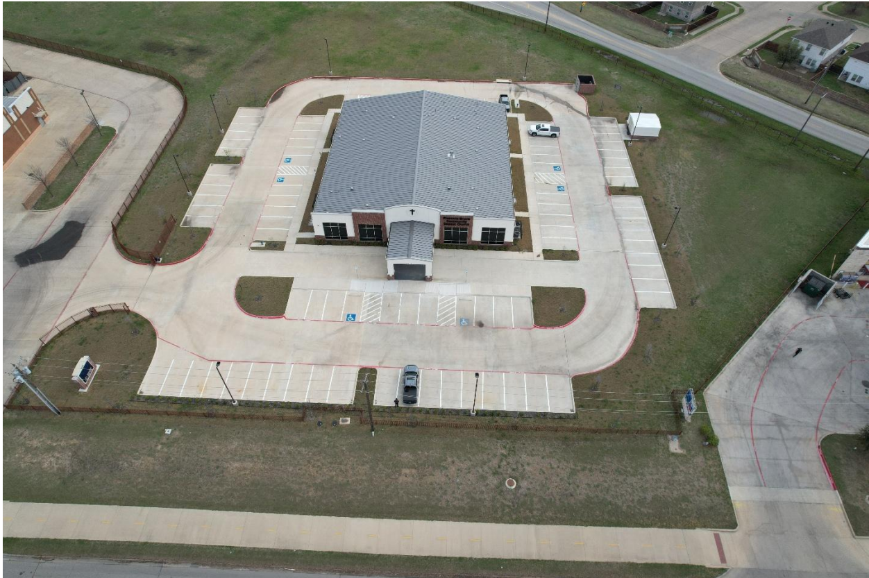
Front of subject property
