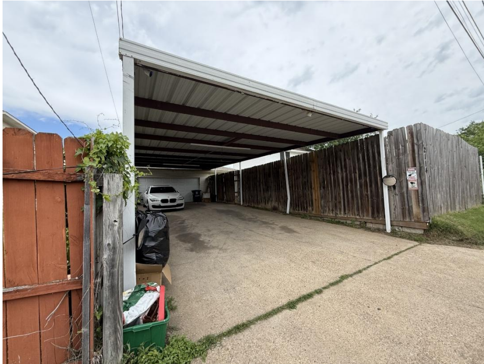
Subject property's rear carport
