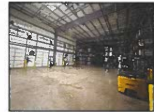
9 Interior Warehouse (1) SCALE NTS
