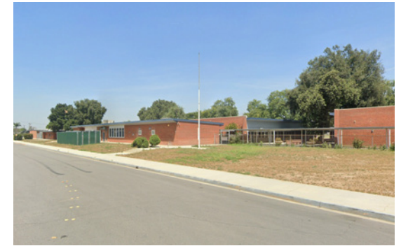
Existing W Del Norte Street and school site buildings; Specific plan area is to the right.
