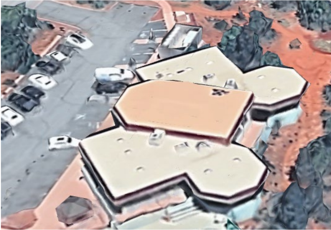
Figure 6 Existing Posse Grounds Building Roof- Aerial view
