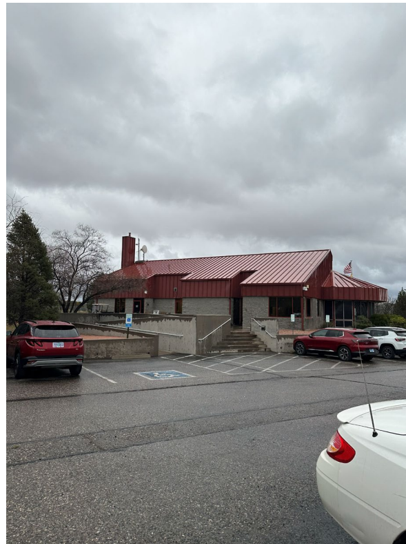
Figure 2 Existing WWTP admin building with red roof
