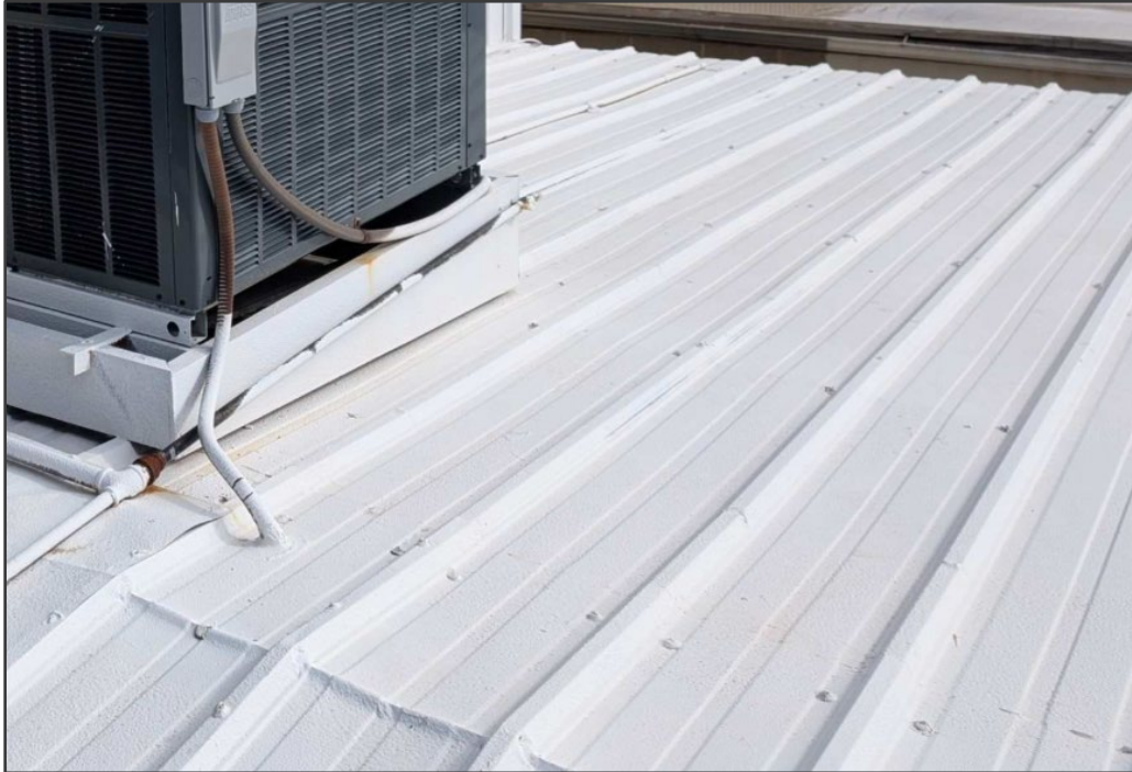
Figure 15 Existing Metal Roof with White Coating
