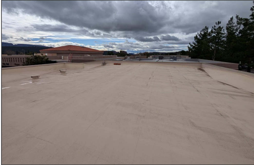
Figure 19 Existing City Hall/Police Department Building Roof
