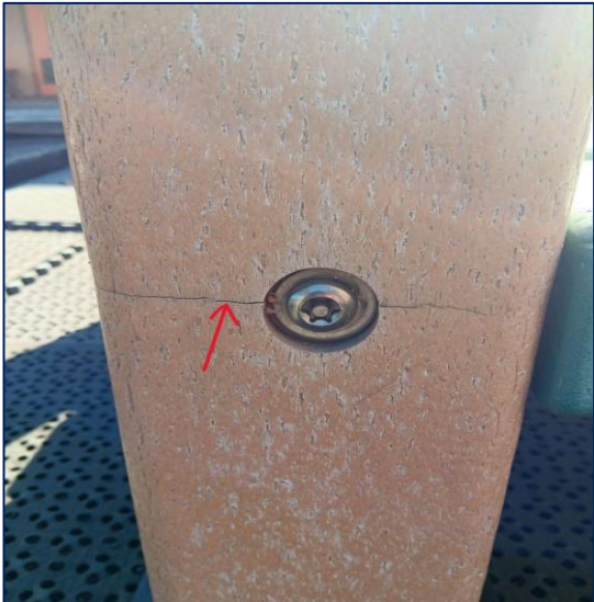
Structure cracked in multiple areas. Currently closed from use.
